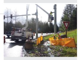
Traffic control measures, like the barrier cones used in this picture, can prevent motor vehicles from coming into contact with elevating work platform.
