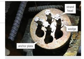
This photo shows 4 strand "heads" held in tension by embedded wedges. Wedges were burned out of the 3 empty holes at the bottom of the plate, allowing the strand heads to pull back into the structure behind the anchor plate so they are no longer visible.
