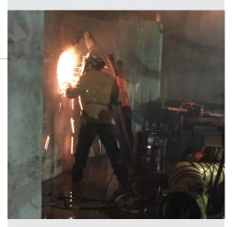
Caution! Ventilation setups like this aren't enough. Better local exhaust ventilation (LEV) options are available like portable equipment used in welding environments.
