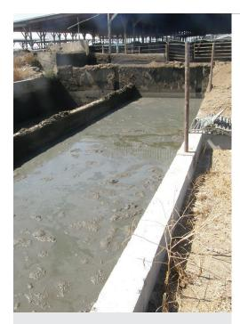
Danger, drowning hazard! All it takes is a stumble on uneven ground or getting struck by moving equipment to launch a worker over the edge of manure separator lagoon like this one. When this is possible, proper railings or barriers can keep workers safe and working.
