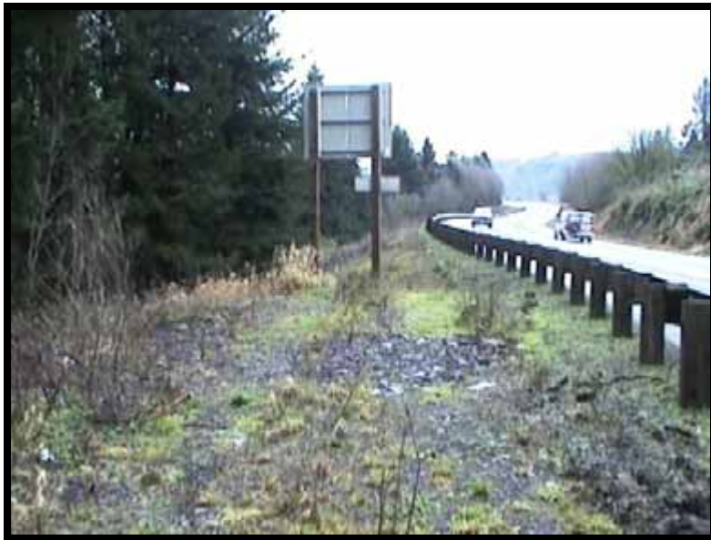
Photo 6: AFTER – Shows the work zone site during 2nd post-incident FACE investigation site visit, and after fill, rock and gravel had been brought in so sign installation could be completed off the roadway without impacting highway traffic. This view is looking east along the westbound lane of highway.
