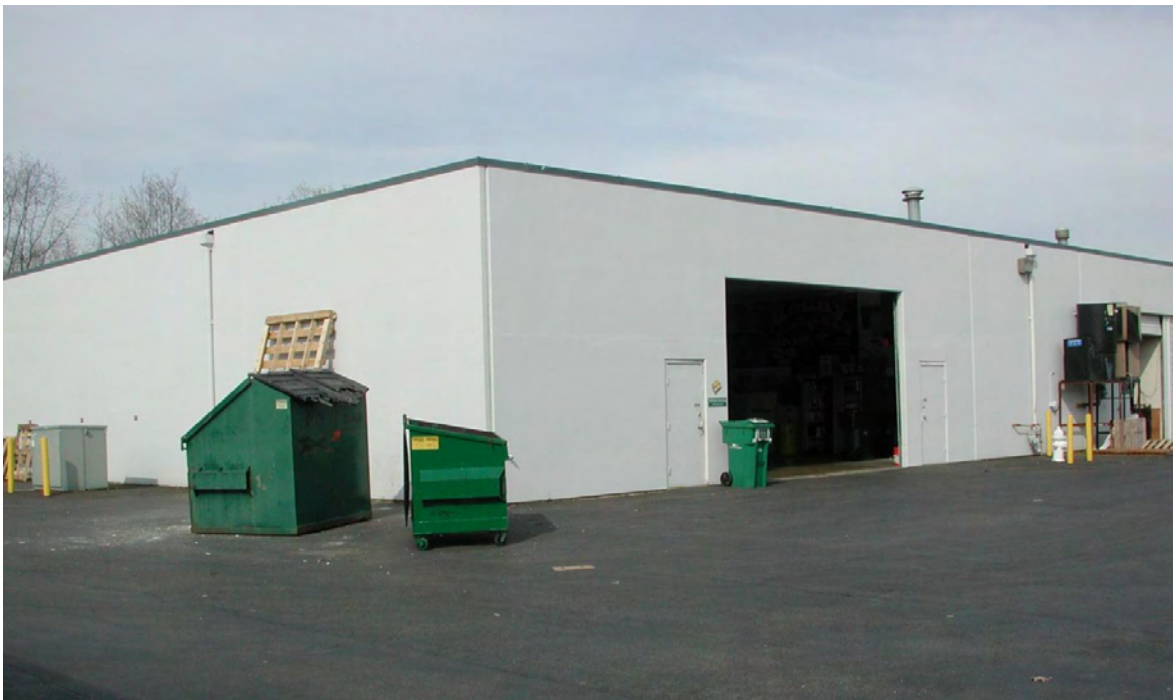
Photo 8. Incident location warehouse (victim accessed the warehouse and its office space through this door).
