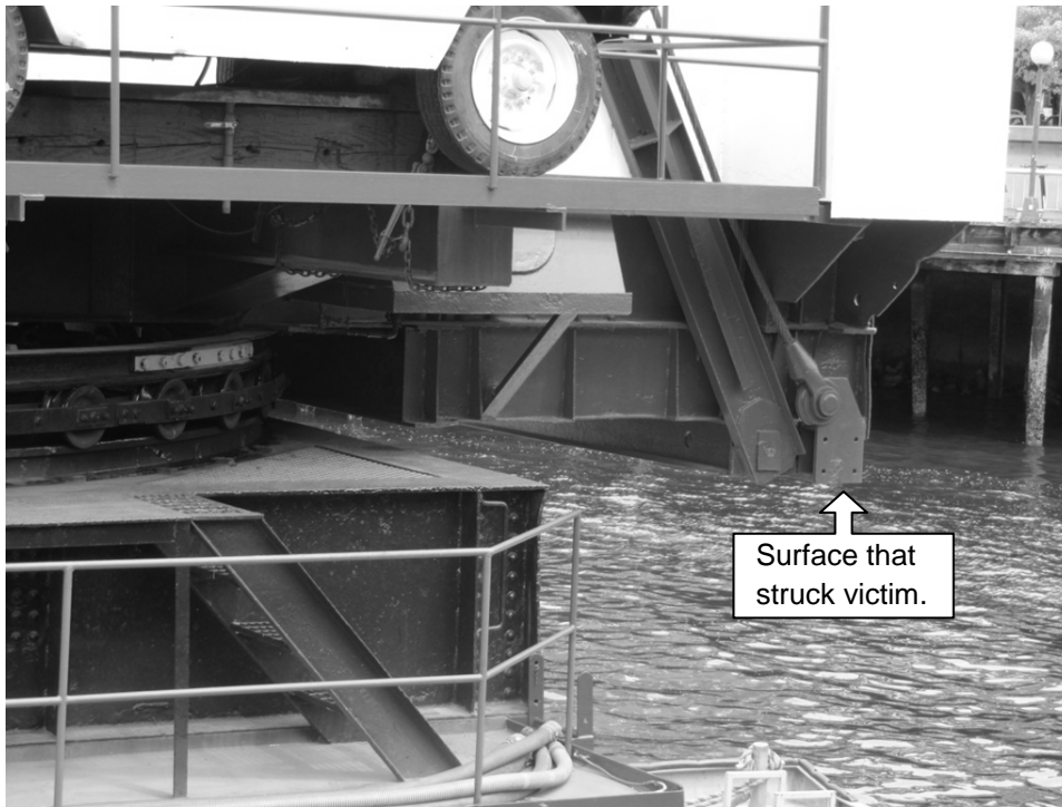
Photo 5: Crane counterweight which struck victim (photo taken shortly after incident).
