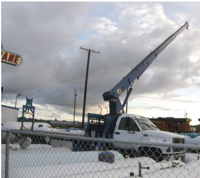
Photo 1. 8-ton boom truck crane with telescopic boom extended at incident site in employer's propane tank storage yard.
