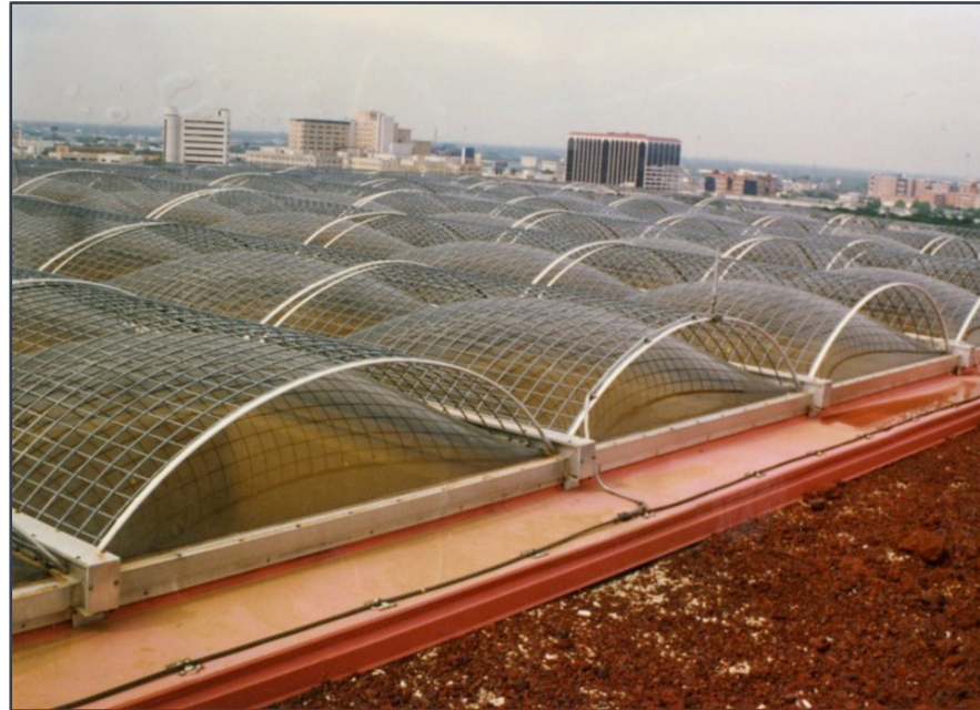
Example of skylights guarded with screens.
