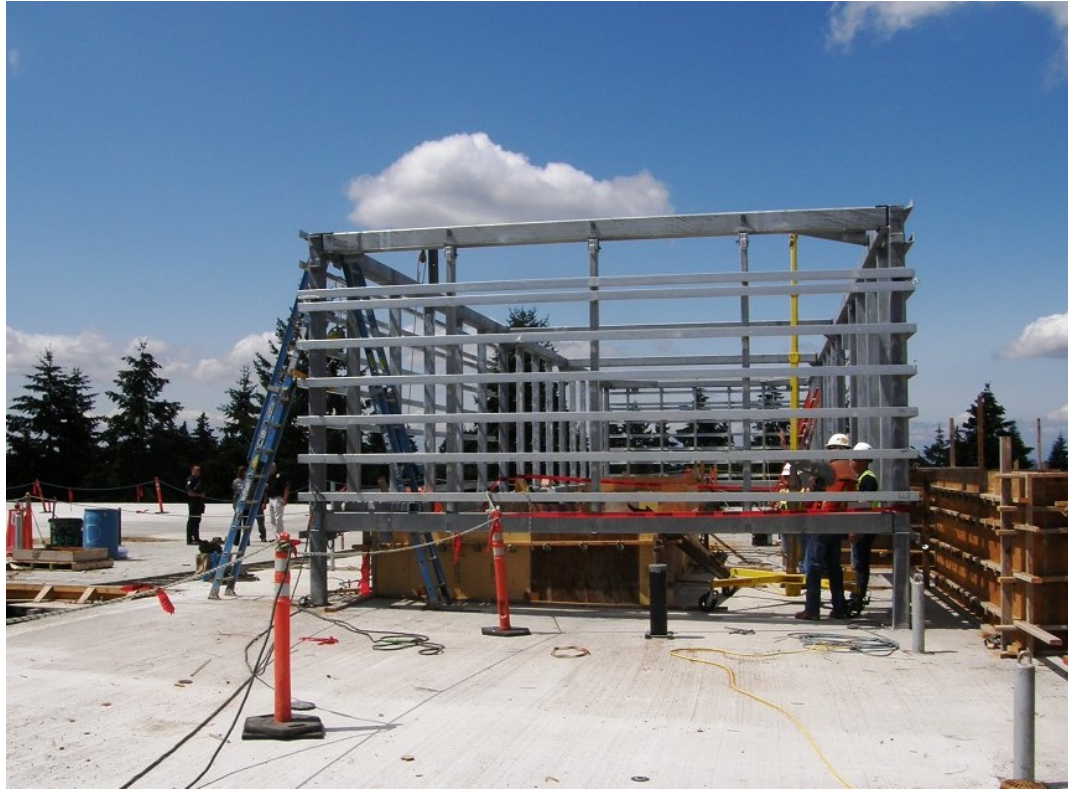
Photo 1. Incident scene showing rooftop windwall structure.
