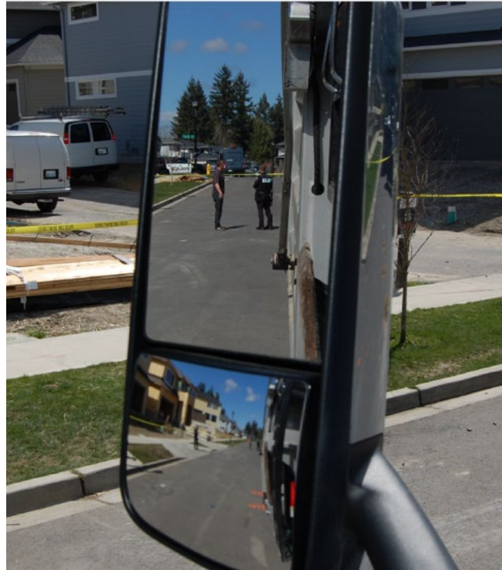
Photo 3. View of incident scene in dump truck's side view mirror shows workers are difficult to see if not wearing high-visibility vests.
