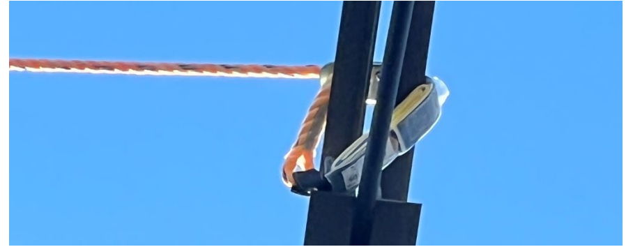
Photo 6. Vertical lifeline wrapped around beam and connected to itself.
