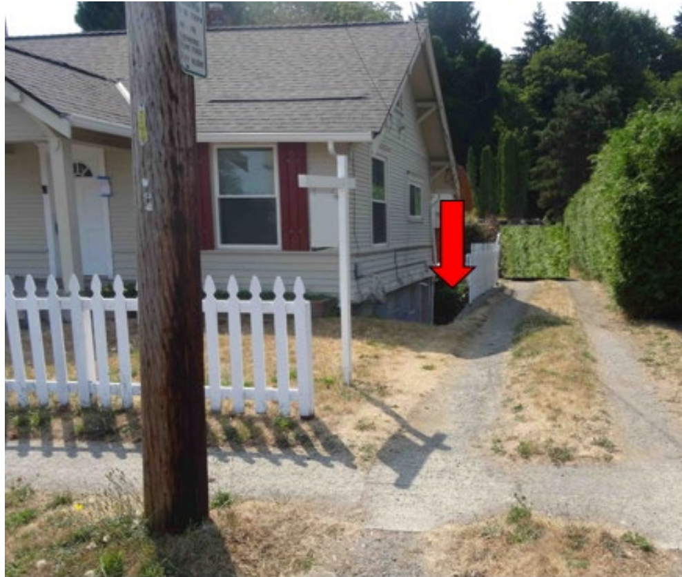
Photo 6: View of incident scene from road. Arrow points to basement entrance area where the lone worker fell from the ladder.
