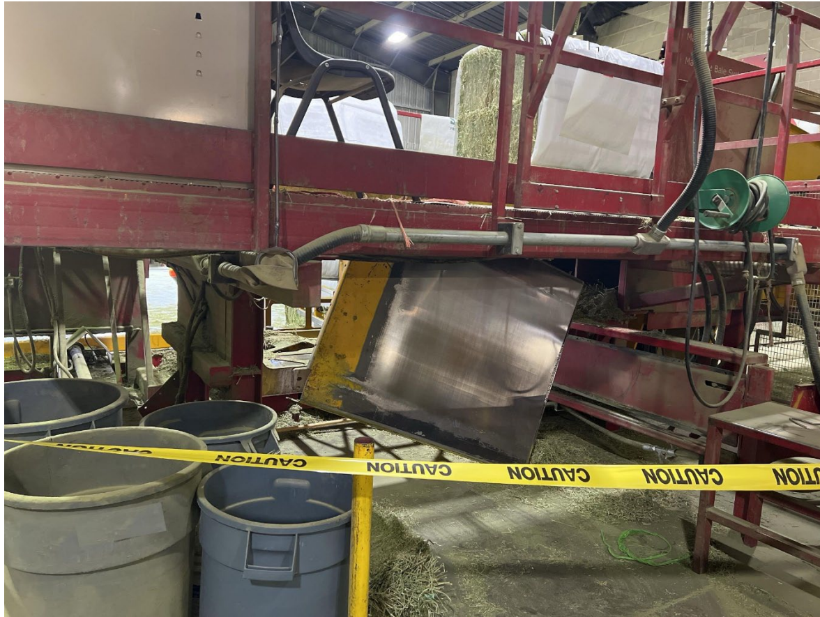
Photo 3. Unguarded area behind hay bale elevator where worker entered before being crushed. Note lack of hazard warning and LOTO procedure requirement signage.
