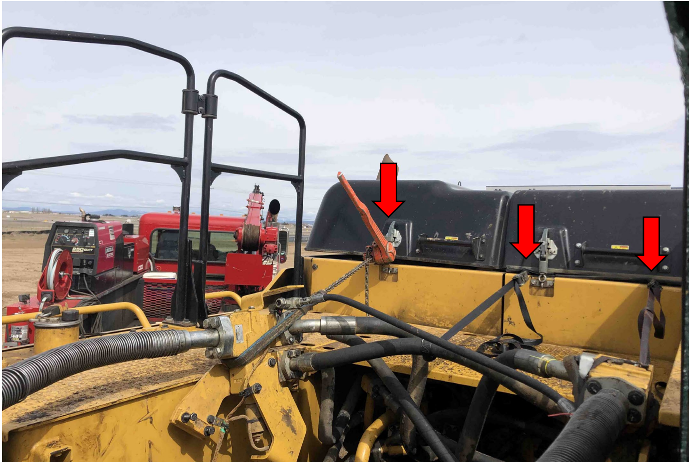
Photo 4. Arrows show how ratchet straps and a come-along pose trip hazards on the platform around the swing drive compartment.
