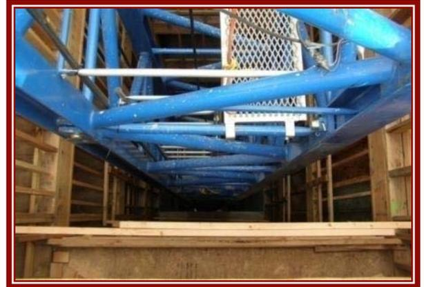
Incident scene showing the elevator shaft and crane mast with its ladder and a landing. The victim fell into the shaft outside of the mast structure, apparently while trying to exit the mast and gain access to the 6<sup>th</sup> floor of the building.
