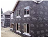
Residential Window Installation
