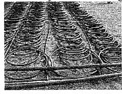
Loop field for a 12-ton system (unusually large for most residential applications)
