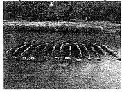
12-ton pond loop system being sunk to the bottom of a pond Slinky closed loop field
