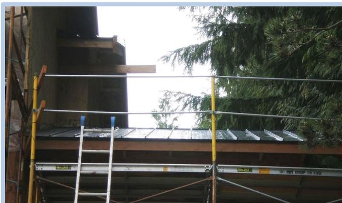
Photo of incident scene showing the sheet metal roof from which the roofer slipped and the scaffold deck he then rolled off and fell 20 feet to the ground.
