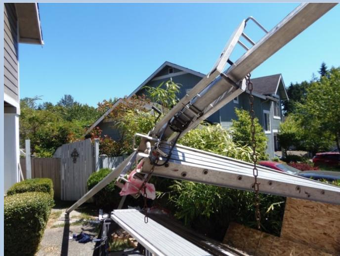
Photo of incident scene with collapsed aluminum three pole pump jack scaffold.
