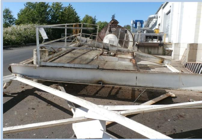
Incident scene showing the collapsed steel structure that struck the victim during demolition. The victim was struck by the steel beam in the center of the photo.
