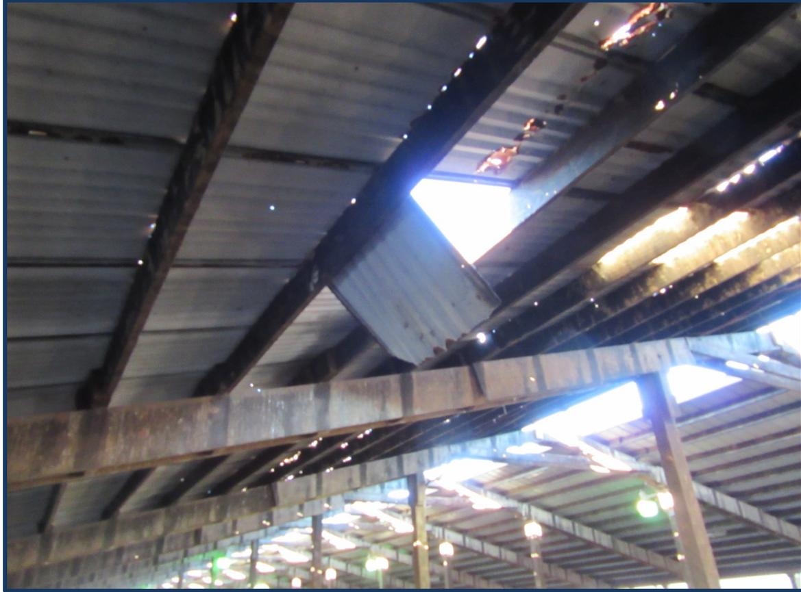
Incident scene showing part of the cow barn metal roof that gave way when the victim stepped on it and fell through, landing 12 feet below.
