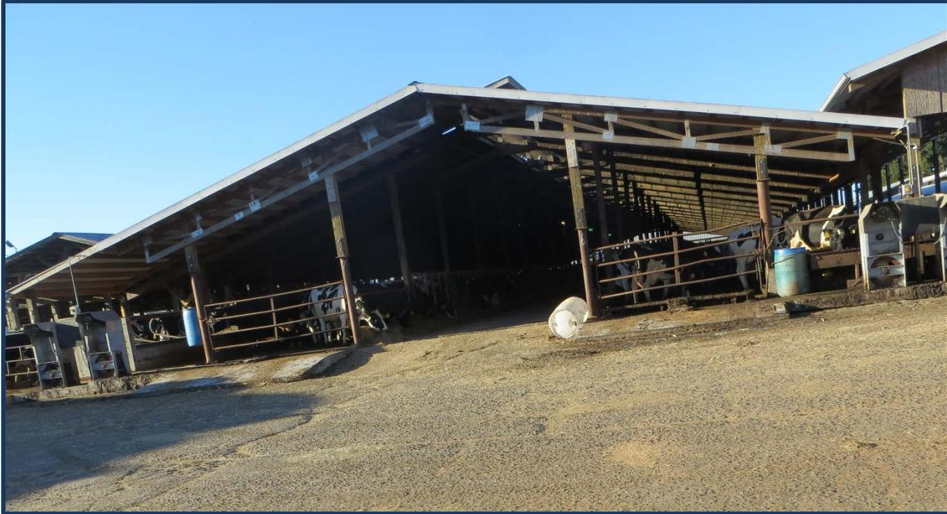
Incident scene showing the cow barn. The victim stepped on a portion of the metal roof and it gave way and he fell 12 feet, landing on concrete.
