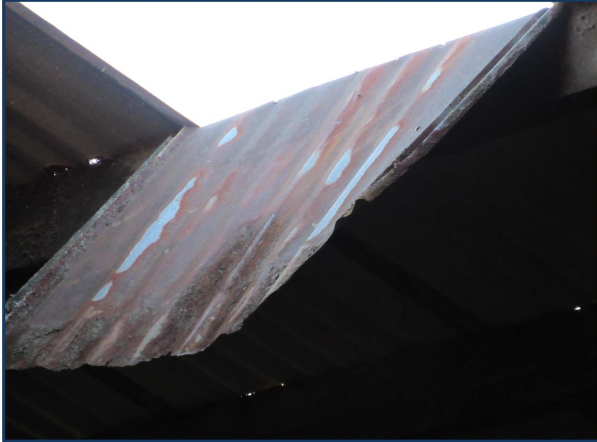
Section of metal roof that gave way when stepped on by the victim.
