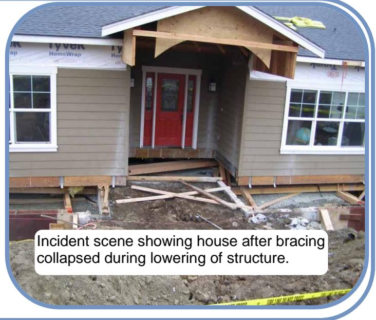
Incident scene showing house after bracing collapsed during lowering of structure.
