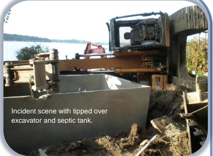
Incident scene with tipped over excavator and septic tank.
