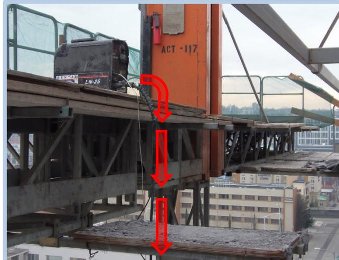
Incident scene showing the mast scaffold platform where an ironworker who had disconnected his fall protection was walking and tripped over a welding cable and fell 72 feet.
