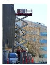
Incident scene showing the scissor lift from which the laborer fell 60 feet.
