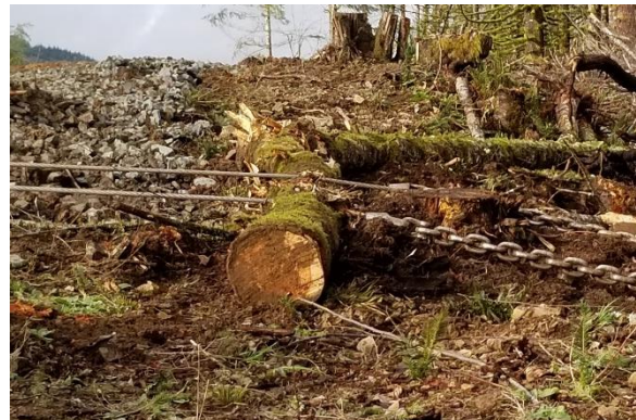
Photo 4. Logs placed to keep lines from rubbing against rocks on road.
