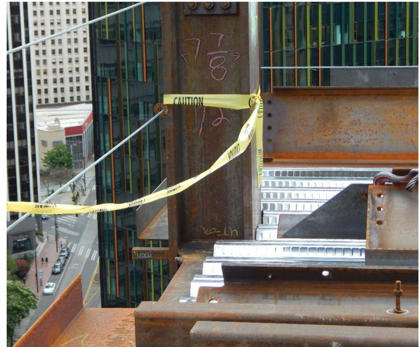
A 29-year-old ironworker was severely injured after falling through a bent plate gap and landing 80 feet below in a debris net.
