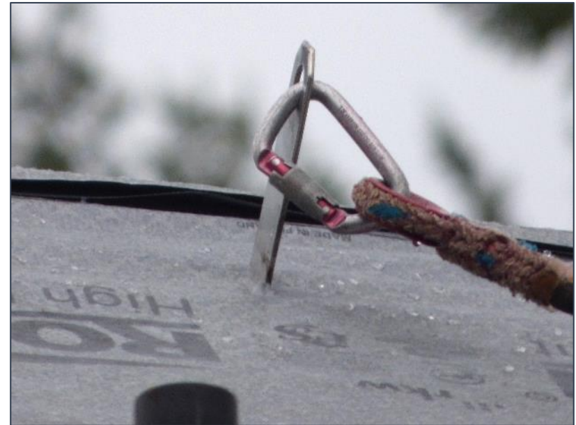
Photo 3. Close-up of the anchor.
