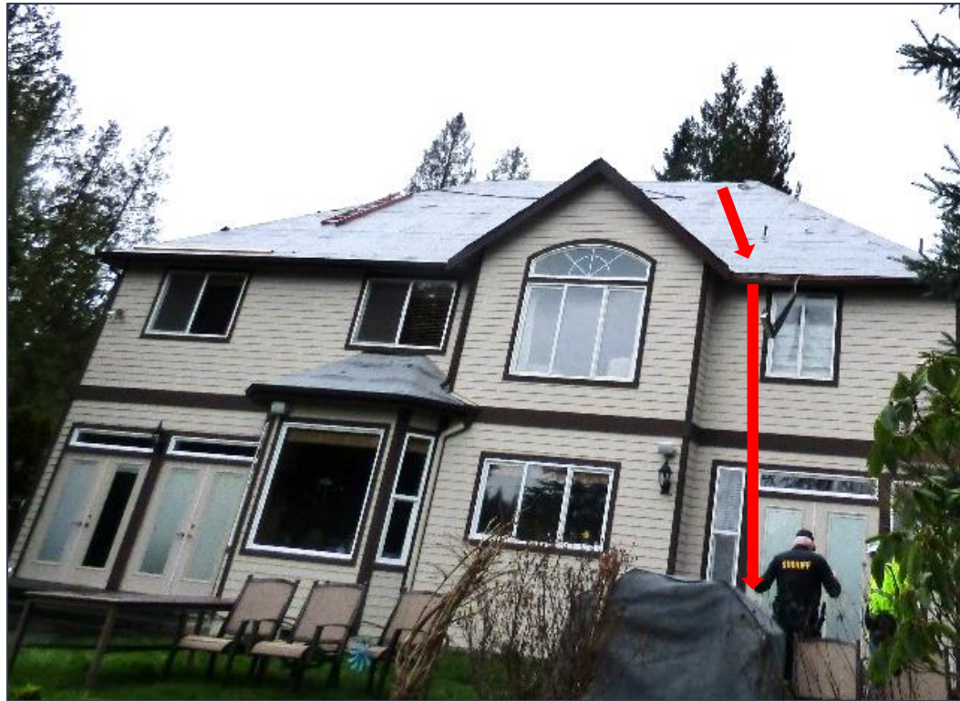
Photo 1. Incident scene showing where the roofer slipped and fell.
