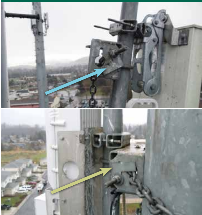
The green arrow shows the correct installation of a chain mount box. The blue arrow shows the chain mount box that failed (it was installed upside down.)
