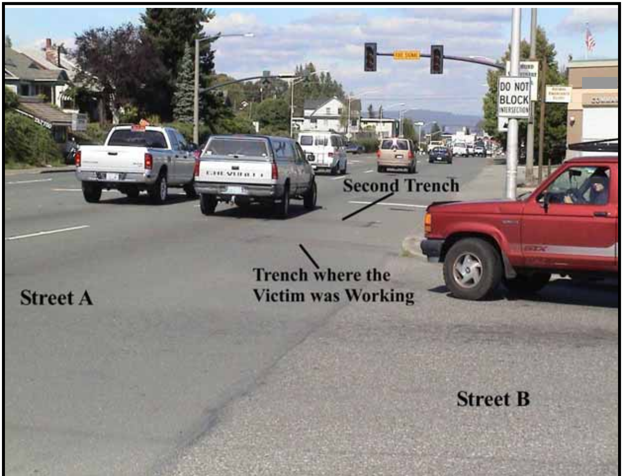
Photo 2: Shows the work zone incident site after project completion, and the intersection of streets (A) and (B) Near the work zone. The photo also shows the close proximity to traffic. The area in front of the trench and the area where the red pick-up truck is located were coned off to traffic (looking north).
