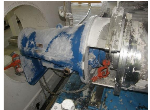
Photo 4 “Come-along” lever pullers attached to recirculation pump.
