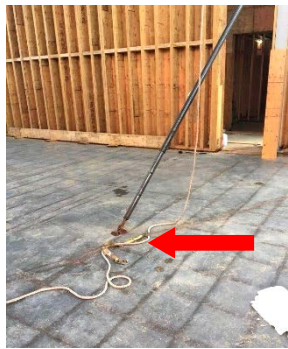
Rope grab showing slack in lifeline.
