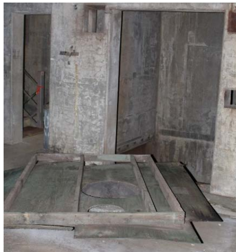
Photos 5, 6, and 7: The left photo shows elevator shaft with plywood guard down. The center photo shows the plywood guard resting on the round opening frame built into the guard. The right photo shows bottom right corner of guard with area that appears to have been recently splintered.
