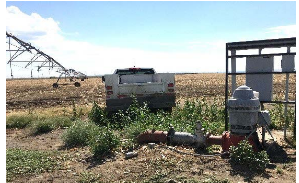
The operator backed into the system's water main, breaking off its flow regulator and pressure switch. This caused water to be released. The operator was electrocuted when he picked up the electrified switch.
