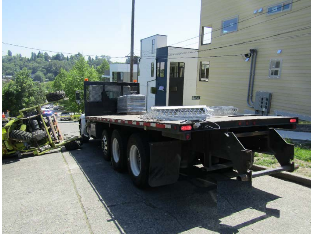
Photo 3. Delivery truck with overturned forklift on city street. The driver was using the forklift to lift a pallet of paving blocks from the flatbed when the forklift overturned.
