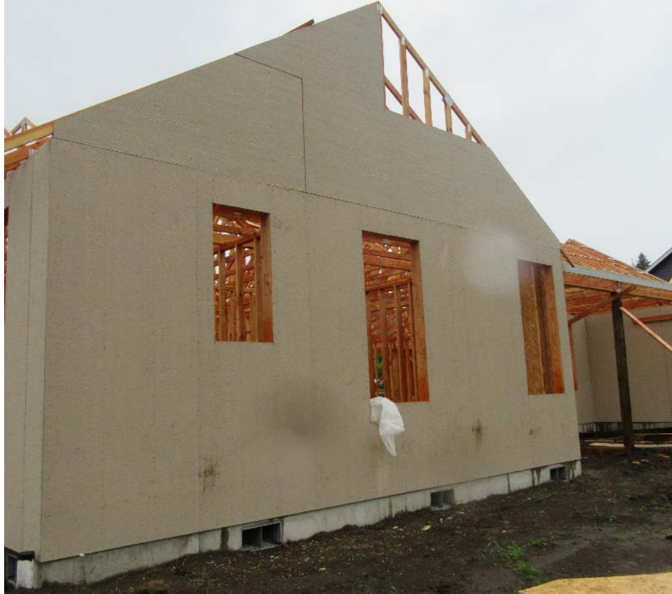
Photo 1. Side of house where framer placed an extension ladder on soft, uneven dirt. As he was climbing, it shifted and he fell eight feet.
