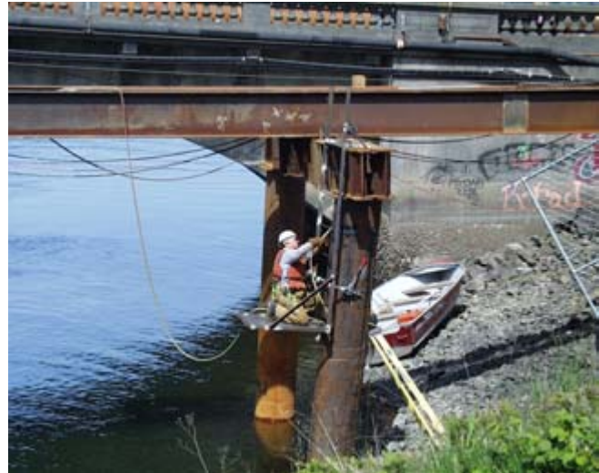
Worker wearing PFD, eye protection, hand protection, and head protection while welding.
