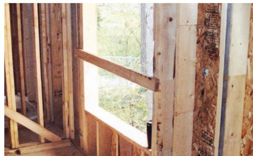
Guardrails are required across openings that have sill heights less than 39 inches.
