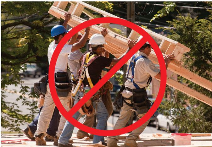
Workers are exposed to falls while raising a wall without using fall protection. Workers will also be exposed to falls through the unguarded opening once the wall is anchored in place.
