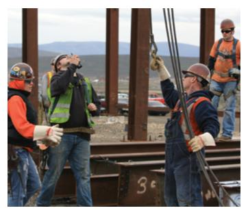
Material handling presents many hazards on the construction job site. In particular, an incorrectly rigged load can lead to falling material, property damage and equipment failure or tip over.
