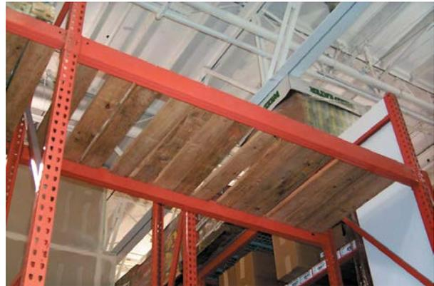
Check that wood stringers or decking in racks are in good condition. They may not support the load if the pallet is not properly placed on both front and rear rails.
