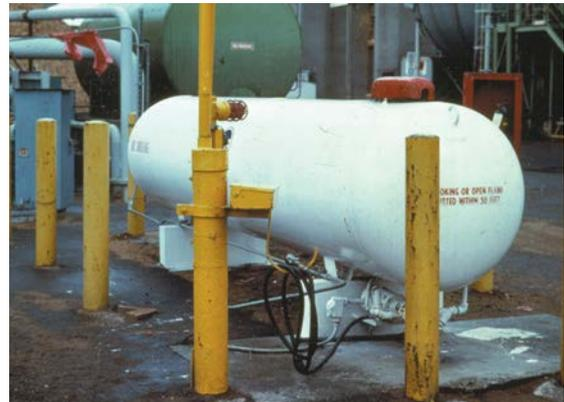
Propane tank used to refill the forklift LPG tank is protected against vehicle damage by heavy posts and must be well ventilated and not near any ignition sources.
