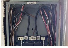
**Picture of the Month:** *If viewing this document online, click on the picture to open a larger image.* This panel had been changed out before the current owner purchased the home. There is no conduit system for the service entrance conductors and no main bonding jumper.
