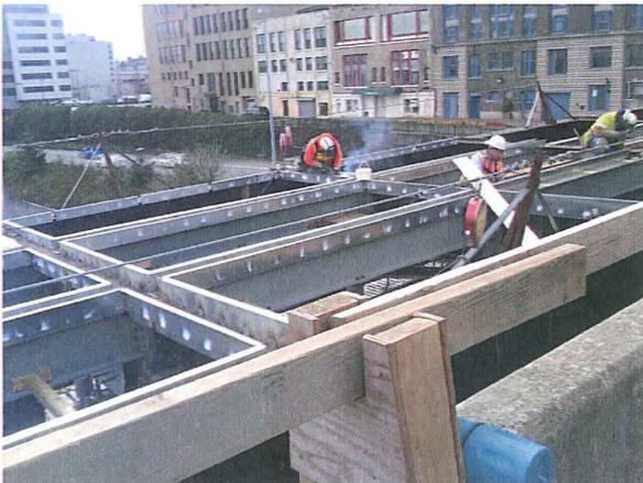
Following welding in place of the edgeforms, corrugated steel sheet decking SIP forms are screwed down onto the welded in place edge forms. Although I didn't get to see workers attaching the deck forms onto the edgeforms during my visit, many forms had been screwed into place and I was able to walk onto and view them closely.
