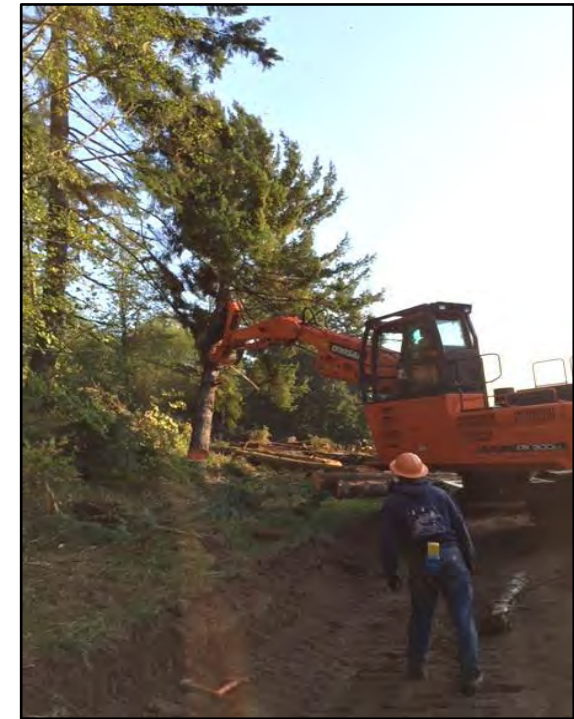
*Cutter safely in the clear while machine pushes tree
