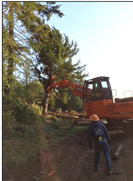
*Cutter safely in the clear while machine pushes tree
