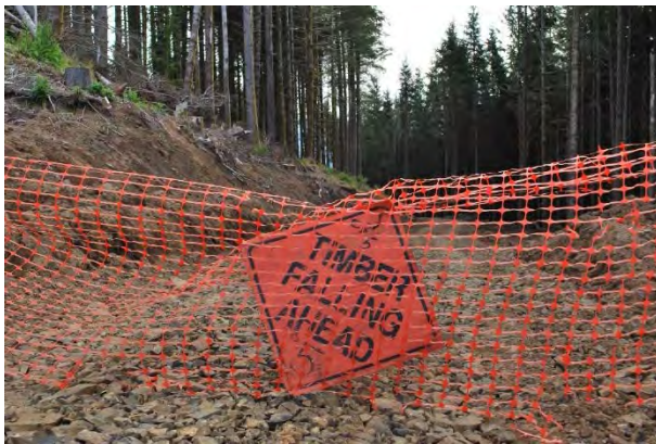
Inform cutters before entering a timber falling area
