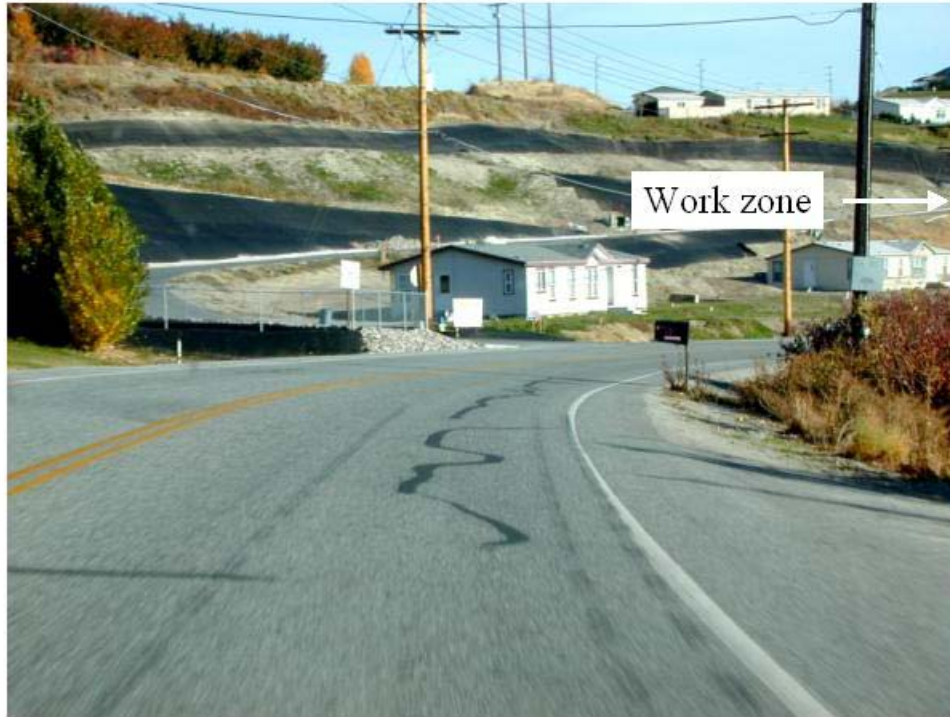
Photograph 1. View approaching the work zone from the south (direction from which the intruding vehicle approached).
