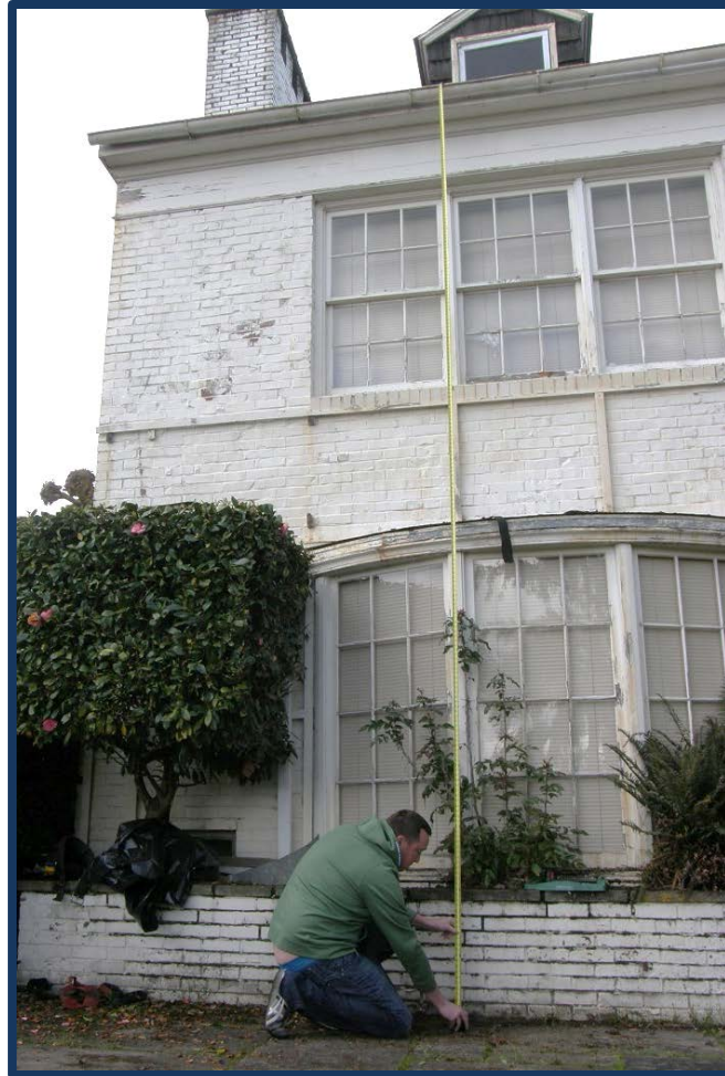
Incident scene showing the location where the roofer fell 19 feet from the roof.
