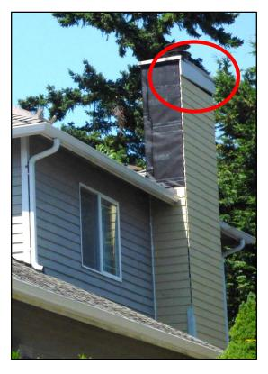
**Photo 4**. The foreman was working from an extension ladder leaned against the chimney chase, using a drill to install a fascia board (indicated by circle). When he reached to his right to put in a second screw, the unsecured ladder slid sideways and he fell.
