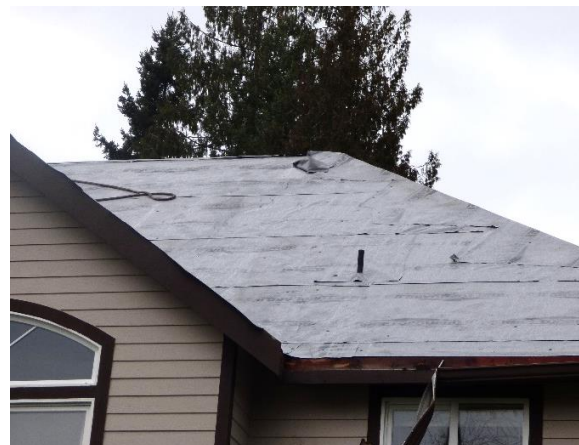
Location where the roofer fell.
