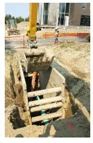
View from excavator cab. The spotter was in the trench to the right in the operator's blind spot.
